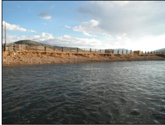
Figure 3.61 – Bank erosion occurring along a fenced ranch property without a riparian buffer.
