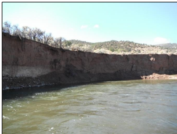
Figure 3.48 – Bank failures were present in some bends along the reach.
