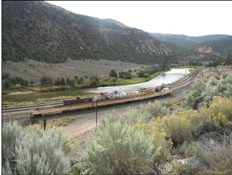
Figure 2.44 – The railroad tracks follow right alongside the river in many areas of the confined valley.
