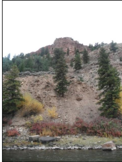
Figure 3.57 – Typical surrounding hillslope in the reach. The highly erodible faces are delivering sediment directly to the river.
