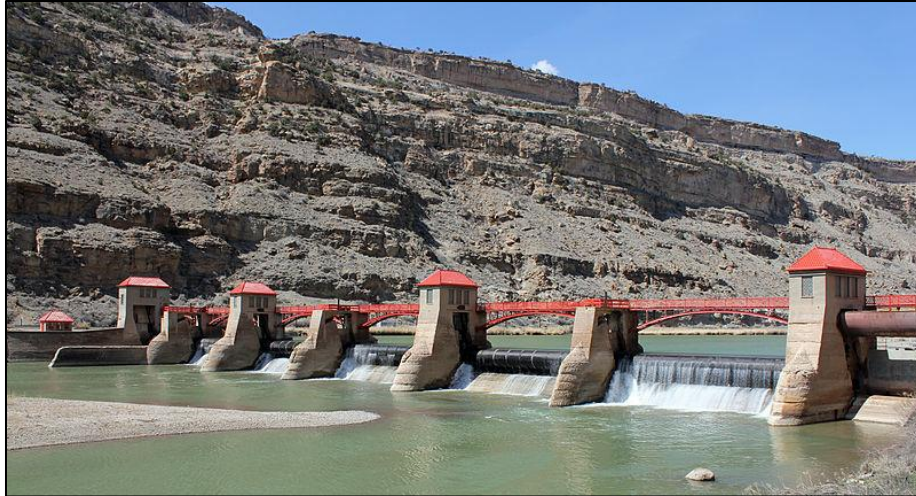
Figure 3.8 – Grand Valley Diversion Dam ( http://commons.wikimedia.org/wiki/File:Grand Valley Diversion Dam.JPG ).
