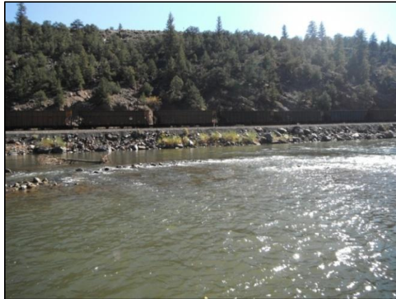
Figure 3.44 – Some willows have established on the riprap banks along the train tracks.
