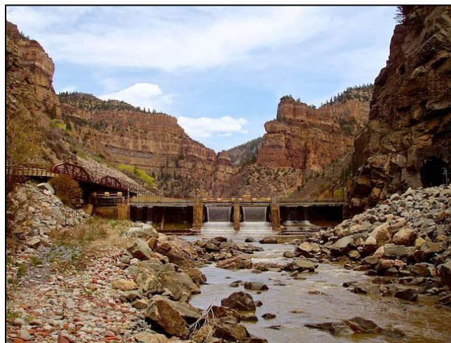
Figure 3.7 – Shoshone Dam diverts water from the Colorado River to the Shoshone Power Plant downstream ( http://krcc.org/post/shoshone-power-plant-big-dog-river ).
