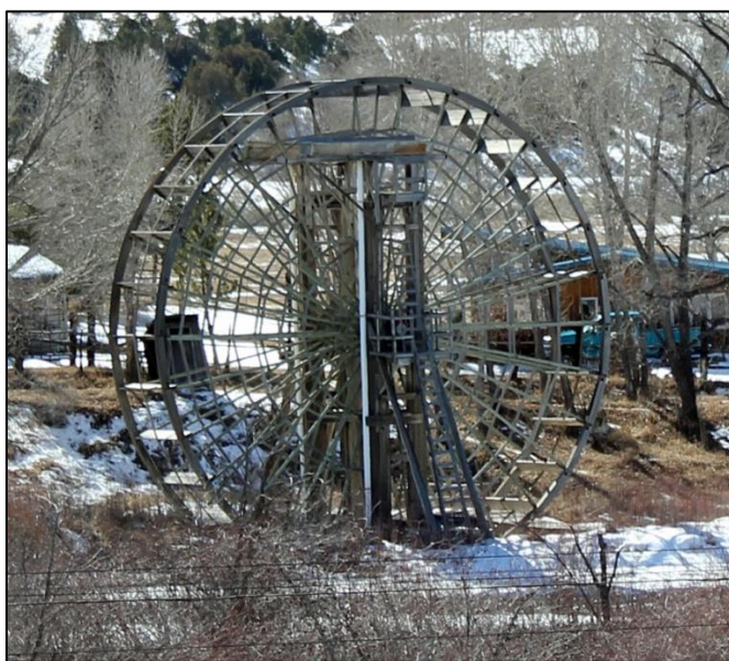
Figure 2.42 – The largest waterwheel in Colorado was built in 1922 just south of McCoy.
