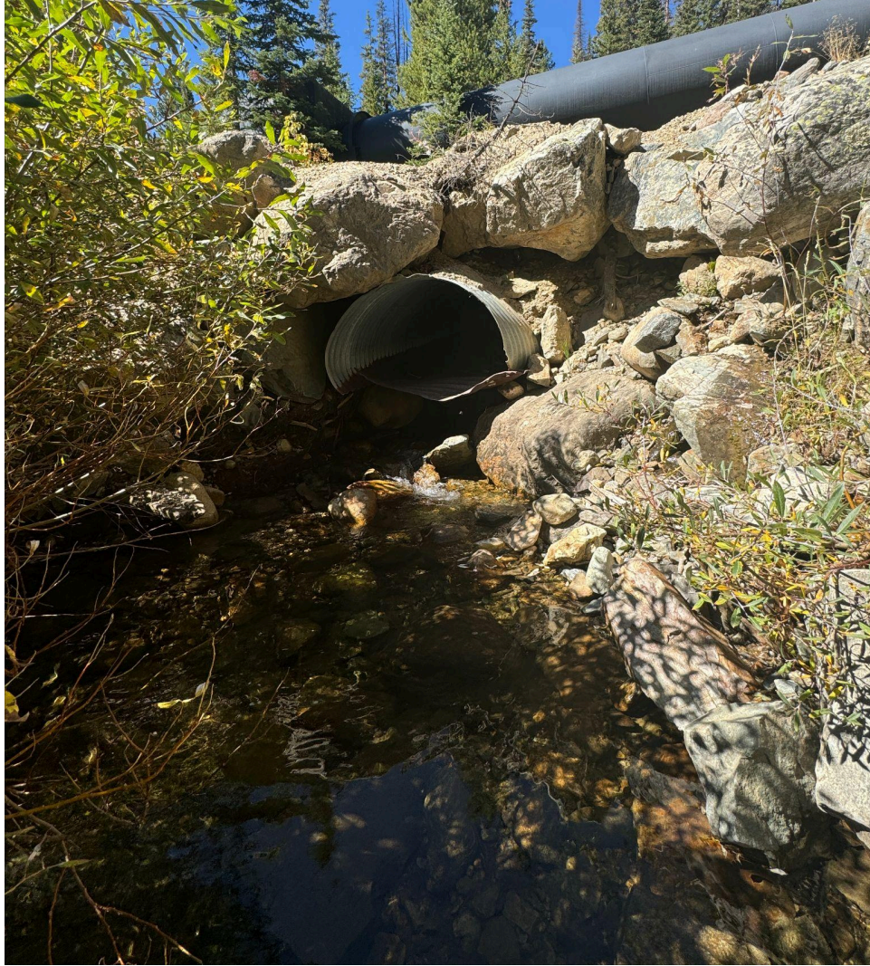
Upper Fancy Stream Crossing; Culvert outflow feeding into a step-pool/cascading system.
