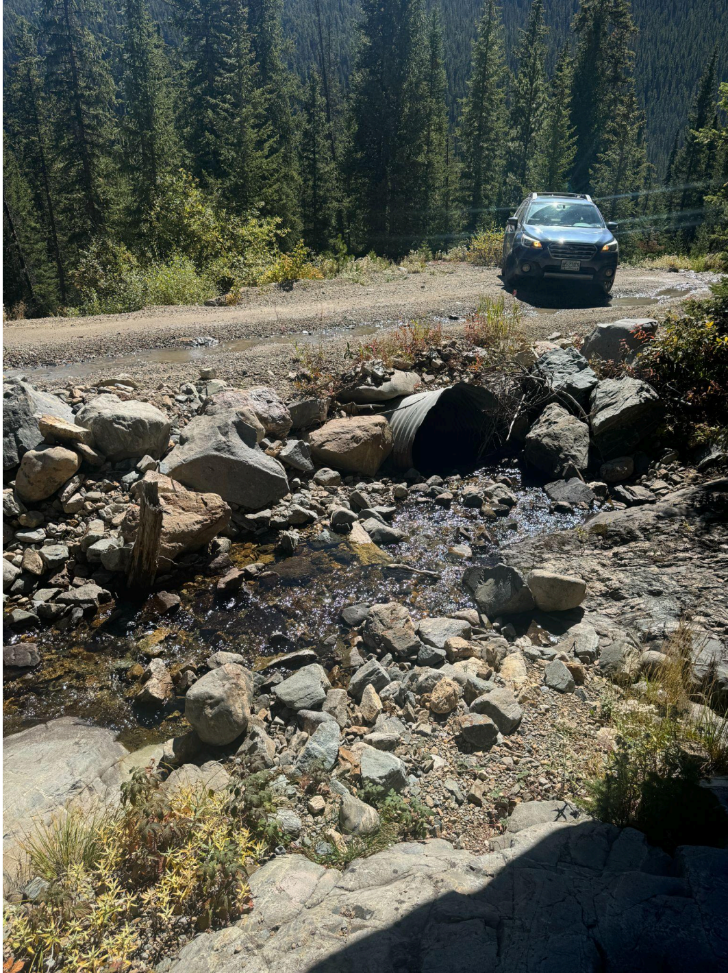
Upper Fancy Stream Crossing; Upstream of culvert. (39°23'42.7"N 106°28'12.9"W)
