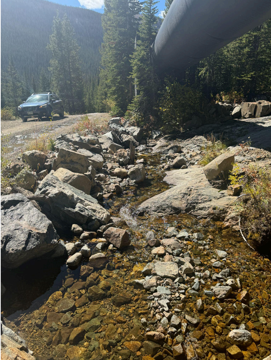
Upper Fancy Stream Crossing; Upstream of culvert facing downstream. (39°23'42.7"N 106°28'12.9"W)
